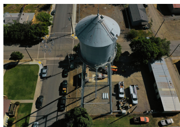
Maxwell Water Tower Railing - 4 Radios
