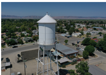
Williams Water Tower Railing - 4 Radios
