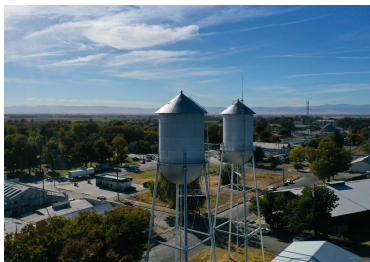
Colusa Reclamation District Tower - 2 Radios
