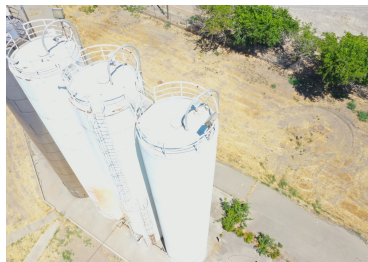
Pirelli Tanks, Colusa 1 Radio
